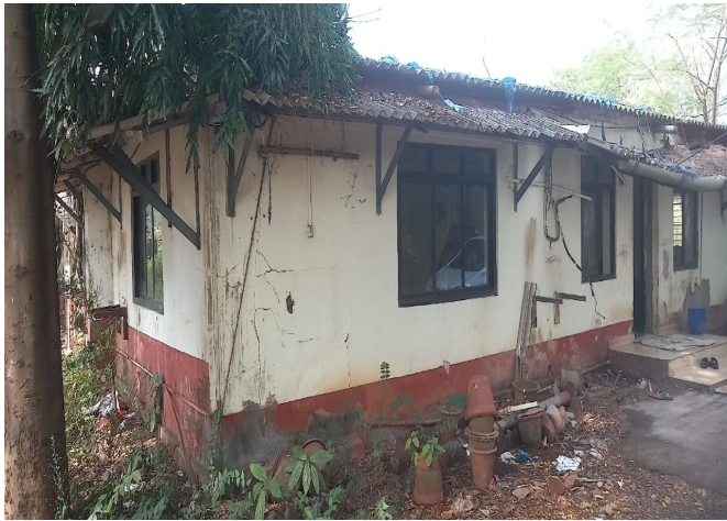
Office Block (Admin Building)
